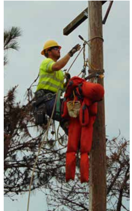
Left: Linemen crew stringing new wire to restore power following December 15 tornado damage. Below: Lineman performing pole top rescue training at safety meeting.
